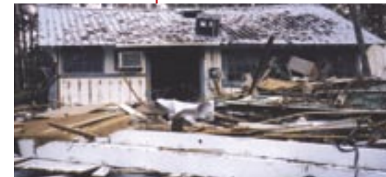
This showroom at Shearwater Pottery in Ocean Springs, Mississippi was one of eleven buildings destroyed beyond repair by Hurricane Katrina. Shearwater was started by the Anderson family in 1928.
